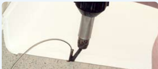
Hot seam weld vinyl flooring directly to the Swifts TRUESEAL2 profile.
